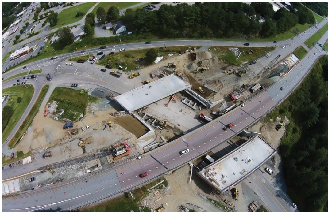
A lateral bridge slide on I-91 in Hartford, Vermont. The study of friction in bridge sliding systems led to recommended design values for lateral slide bridge installations.
